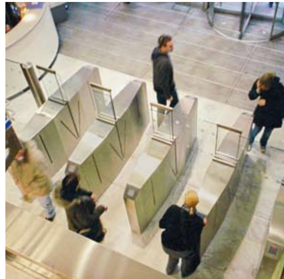
Type and number of turnstile depend on number of visitors and peak times
